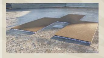
Trace (rake handle, screw driver – can use spray paint) an outline around panels and set panels aside
