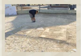
Dig around traced area lines at least 2"- 3" to outside of original traced placement to 'oversize' the hole area... room to adjust Field Armor placement in hole
